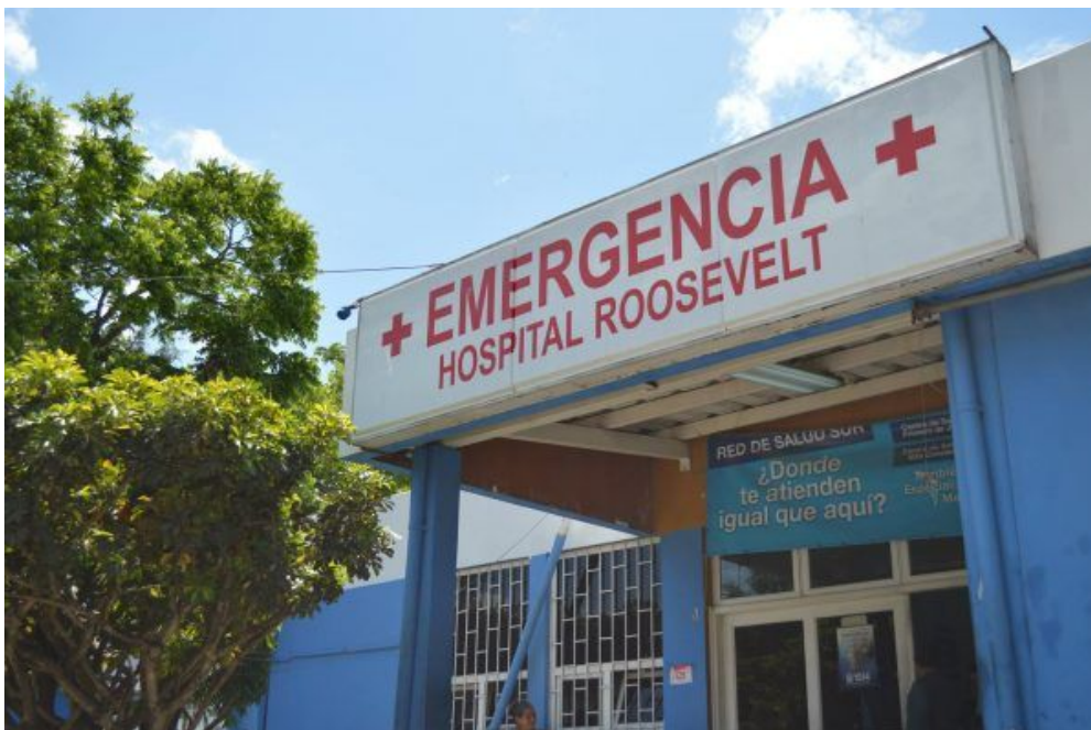
Figure 6 [27] - Emergency Room Entrance
